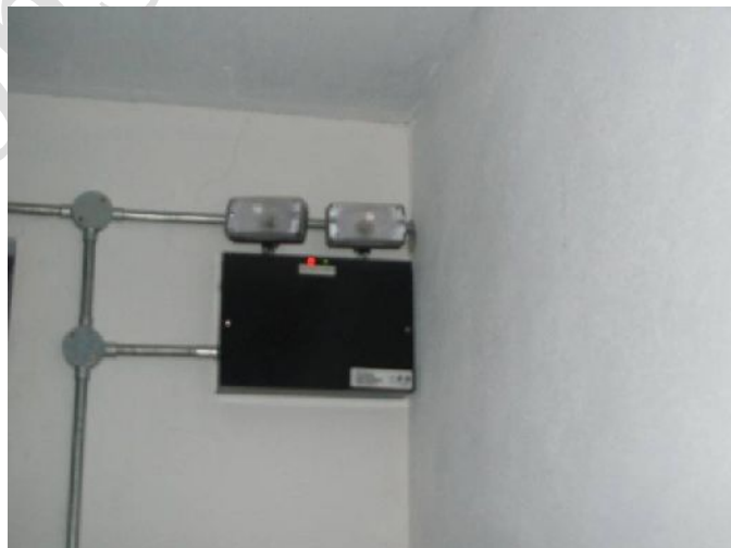
Fig 11.1 Emergency Twin-Spot Fitting in Switch-Room.
