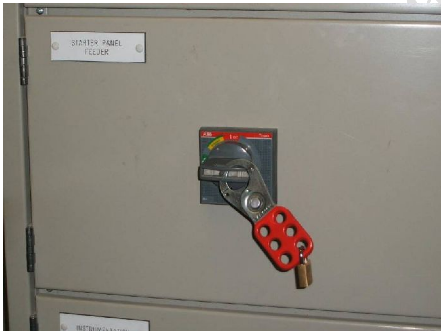
Fig 10.1. Electrical Supply-Isolated and Padlocked “off”
