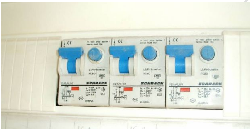
Fig 6.1 Residual Current Devices (RCDs) (fitted to protect socket circuits)
