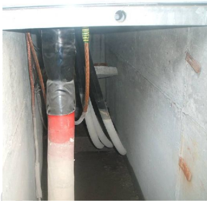
Fig 7.1-Termination of Cables including High Voltage (red) Cable. (Work of this nature will require a high degree of specialist training)
