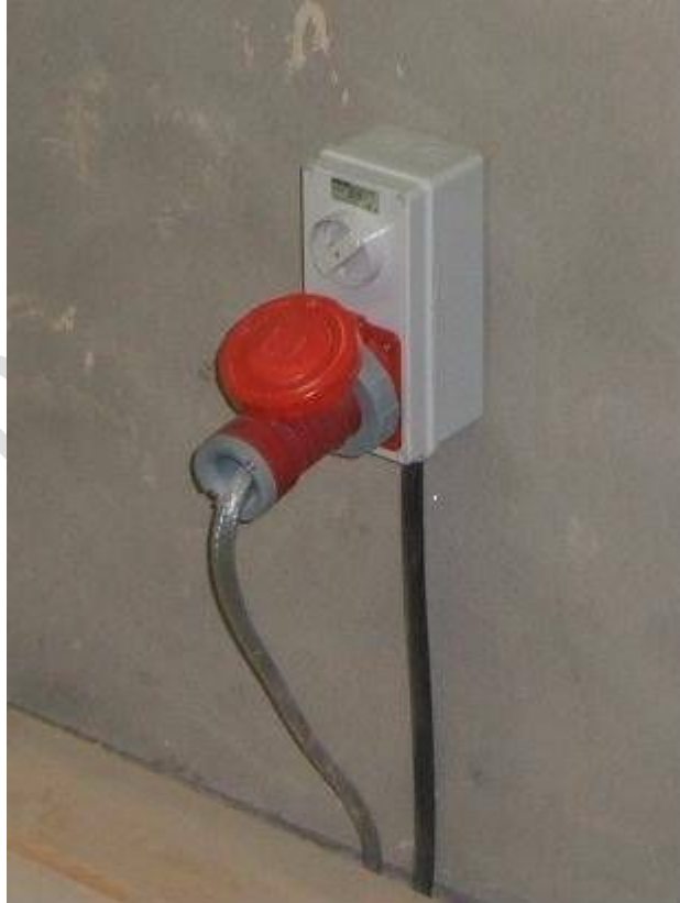
Fig 3.1 Three Phase IP 55 Socket (400 Volt)
