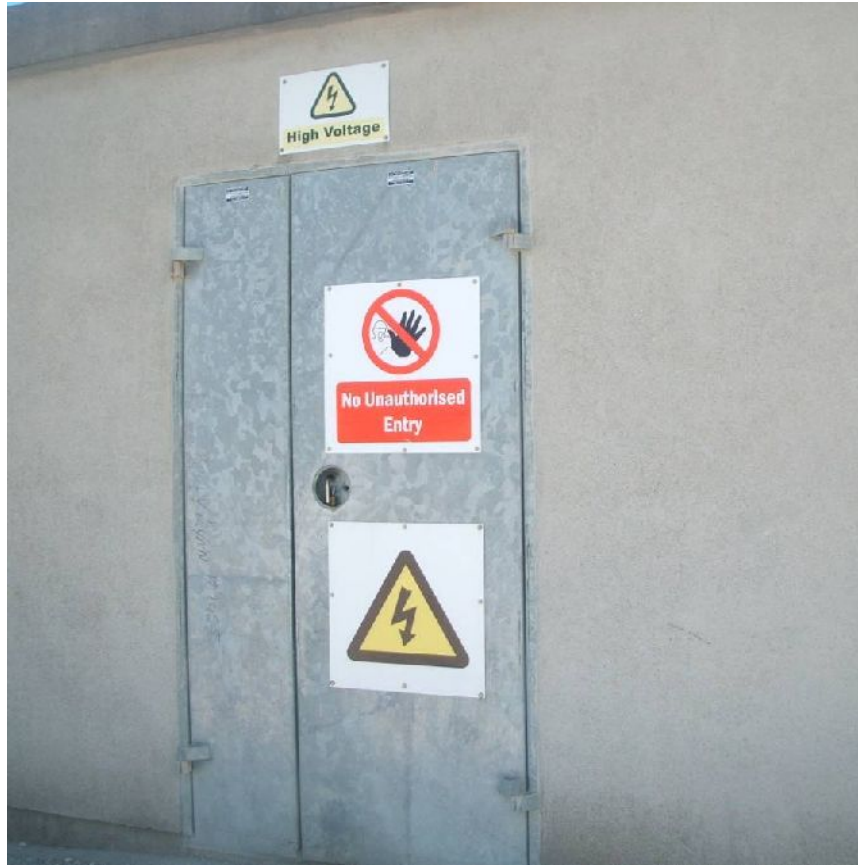
Fig 5.1 Access Controlled to High Voltage Switch Room
