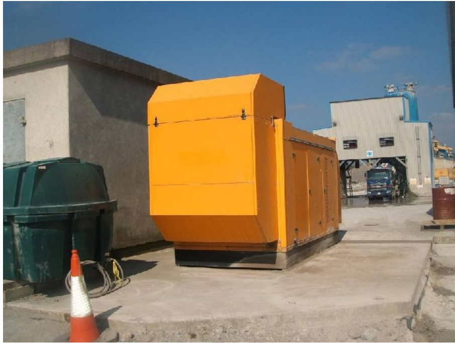
Fig 9.1. Emergency Generator Installation (to maintain electrical supply in the event of a power-cut)
